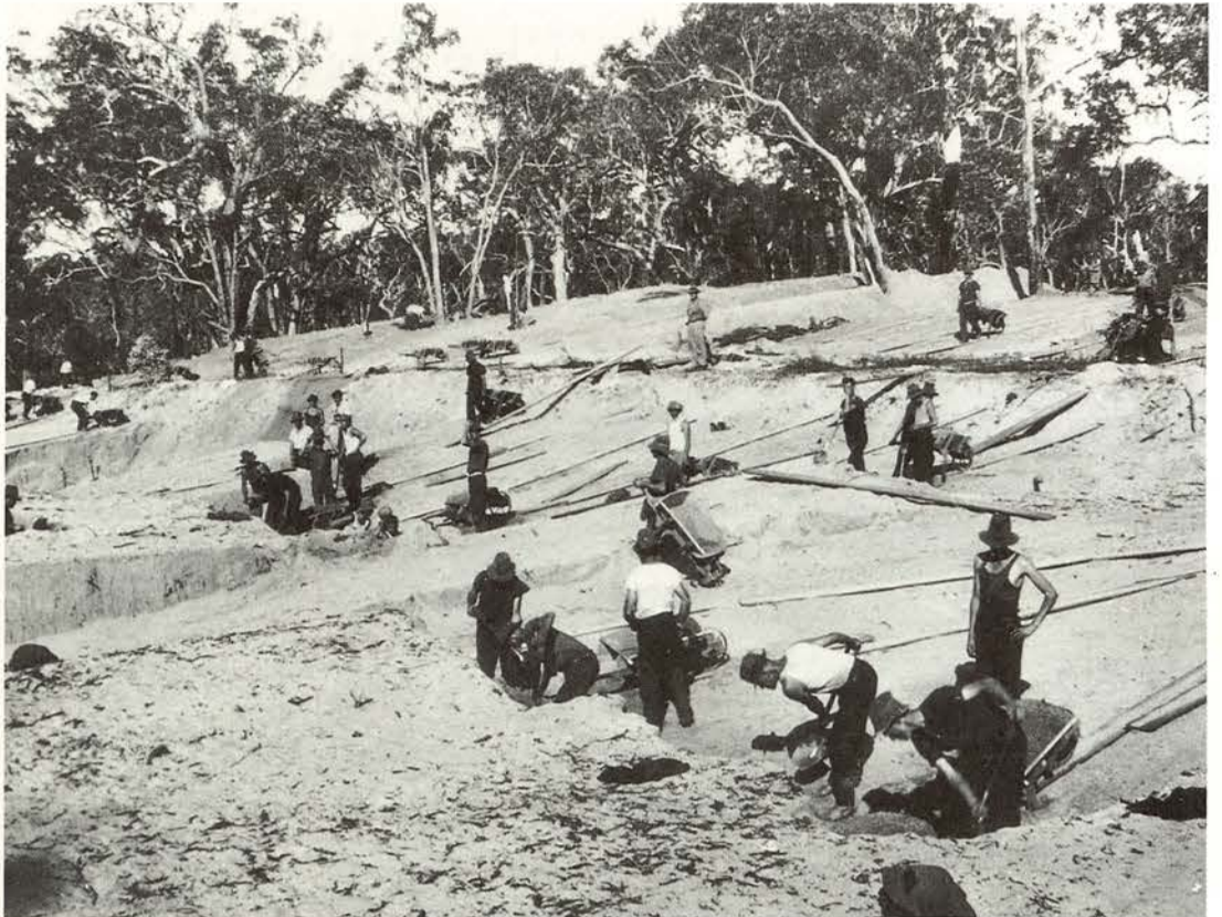
Unemployment relief schemes were introduced in all states during the Great Depression. They were labour-intensive and usually gave immediate benefit on completion. Roads were improved, dams were built and metropolitan sewerage systems were extended. Shown here is the building of the Harvey Dam in Western Australia (photograph c1932). BATTYE LIBRARY
